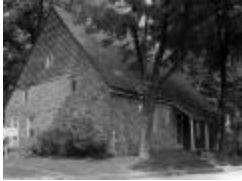
Jean Hasbrouck House in New Paltz, New York (NYS A0245-77_Ulster_B21_14)
