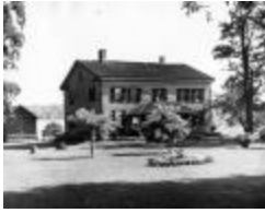
Elmer E. Haller residence in Bennington Center, New York (NYSA_A0245-77_Wyoming_B22_56)
