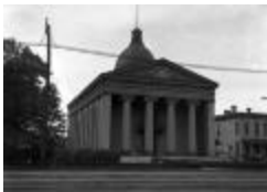
Montgomery County Courthouse located in Fonda, New York. September 30, 1936 (NYSA_A0245-77_Montgomery_B09_31)
