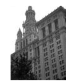
Manhattan Municipal Building in New York City, June 26, 1938 (NYS_A0245-77_NewYork_B09_76)
