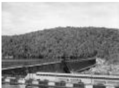
Spiers Falls Power Dam in Glens Falls, New York, 1938 (NYS A0245-77_Warren_B21_63)
