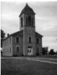
Esperance Presbyterian Church in Esperance, New York (NYS_A0245-77_Schoharie_B20_19)
