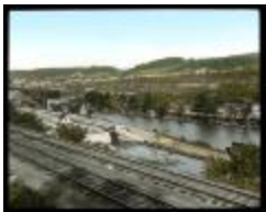
Canal Lock. Little Falls, N. Y. (NYS_A3045-78_X_921_Color)
