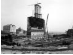
Progress Photo. Construction of Corning Tower. (NYSA_15727_B4_002)
