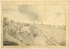
View Showing the Progress of the Work on the Lock Section (NYSA_B0379-85_V17_09-01-1839)
