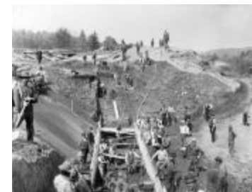
Break in Canal at Forestport, N.Y. (NYS_A0834-77_B5_F16)
