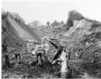
Break in canal at Forestport, N.Y. (NYS_A0834-77_B5_F12)
