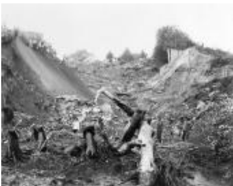
Break in canal at Forestport, N.Y. (NYSA_A0834-77_B5_F12)
