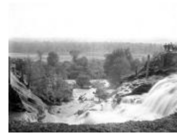
Water rushes through a break in the Forestport Feeder canal levee, 1899 (NYSA_A0834-77_B5_F11)
