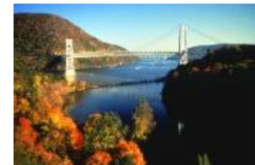
Bear Mountain Bridge across the Hudson, with fall colors (NYSA_B1728-00_B9_D_Slide33)
