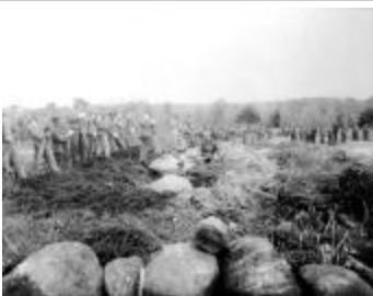
Mental Health Custodial Facilities. Clearing rough land (NYSA_A4228-78_B2_F25_P16)
