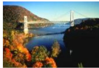
Bear Mountain Bridge across the Hudson, with fall colors (NYSA_B1728-00_B9_D_Slide33)
