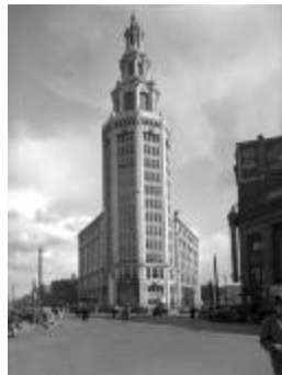
Niagara Mohawk "Electric Building" in Buffalo, New York. October 17, 1937 (NYSA_A0245-77_Erie_B03_50)
