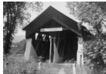
Blenheim Bridge in North Blenheim, New York (NYSA_A0245-77_Schoharie_B20_34_B)
