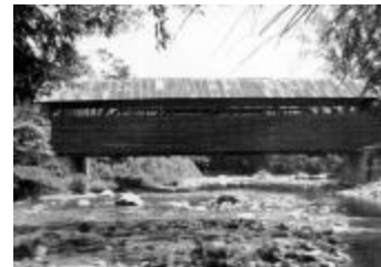
Wagner's Hollow Bridge in Palatine, New York (NYS_A0245- 77_Montgomery_B09_19_A)
