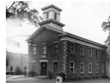
Cobblestone Masonic Temple in Warsaw, New York (NYS_A0245-77_Wyoming_B25_32)
