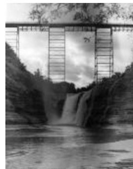
Erie Railroad Bridge over the Upper Falls of the Genesee River in Letchworth Park (NYSA_A0245-77_Livingston_B05_33)
