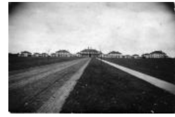
Mental Health Custodial Facilities. Group of Buildings (NYS_A1994-77_B3_F1_P9)
