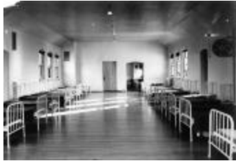
Mental Health Custodial Facilities. Dormitory Infirmary (NYS_A1994-77_B3_F1_P9a)
