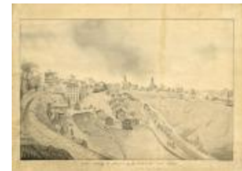
View Showing the Progress of the Work on the Lock Section (NYSA_B0379-85_V17_09-01-1839)
