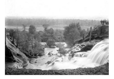
Water rushing through a break in the Forestport Feeder canal levee, 1899. A crowd of onlookers oversee the water to the right. This levee, in upper Oneida County, broke several times over a period of a few years, raising suspicions of intentional sabotage.
