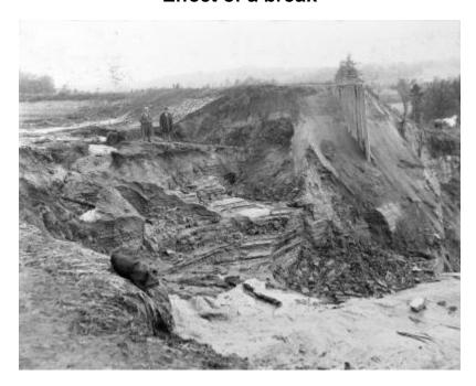
Effect of a break. The men are pictured standing in bottom of canal. In front and below them is chasm torn by escaping water. Heavy timbers used to hold bank firm are shown in section of dike left by torrent.
