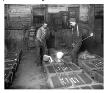
Pouring off stove work with hand ladles, foundry practice; pouring into moulds with hand ladles, (1911).
