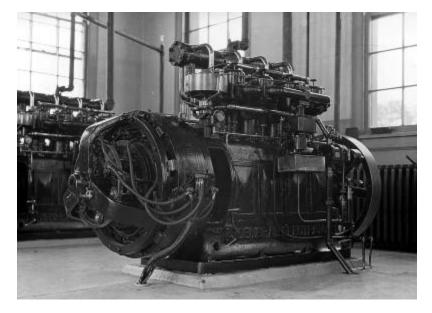
New York. Barge Canal. Dynamos and gasoline motor generator in powerhouse. Tribes Hill, town of Mohawk. (1920)
