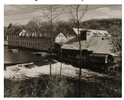
Exterior of large sawmill near Warrensburg in the Adirondack Mountain region, built by Dudley Farlin beween 1818-1820. It was a gang mill containing seventy saws set in gangs. At the time of the photo, the mill was owned by Robert Pasco. The photo was used for an historical feature in one of Hall's Adirondack newspaper publications.
