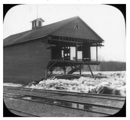
Exterior view of building damaged by ice at Cold Spring along the Hudson River in Putnam County. Much of the walls on at least two sides of the wood framed building have been torn away from the structure. Some of the support beams for the second floor have been dislodged. Huge blocks of ice from the Hudson River are jammed around and under the building. Next to the building in the foreground, a railroad track has been kept clear of ice.
