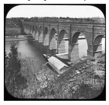
View of High Bridge, a multiple-arch bridge over the Harlem River near New York City. Opened in 1848, the bridge, which runs from Manhattan to the Bronx, is the oldest bridge in New York City connecting two boroughs. It was built to accommodate the Croton Aqueduct, which carried water from the Croton River to Manhattan. The bridge added a pedestrian walkway in the 1860s.
