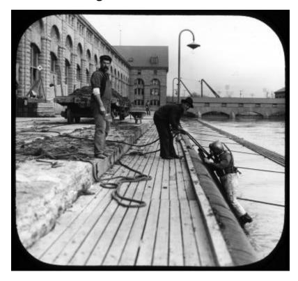
A diver is lowered into the water beside an electric power plant near Niagara Falls. One man looks on while a second man lowers the diver into the water by a rope. The second man also holds onto the air hose running that runs to the diver's helmet.
