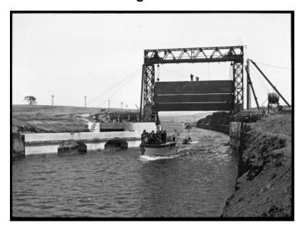
View of the New York State Barge Canal above Crescent Dam, possibly near Lock No. 6 in Waterford, Saratoga County. The slide shows the second emergency dam, or guard gate, being raised, and two motorboats passing by underneath.
