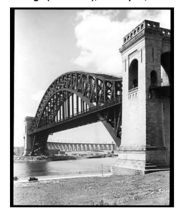
View of the main span of the Hell Gate Bridge, the New York Connecting Railroad's steel arch bridge over the East River in New York City. When the bridge opened in 1916, it was the largest steel arch bridge in the world.
