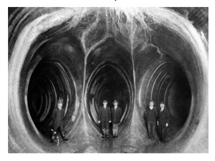
Catskill Aqueduct, showing interior division into three channels for siphon connections. Catskill, from negative of Ewing Galloway, (1923).
