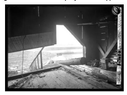
View of a "log jack," a conveyor belt for logs, carrying logs into a sawmill owned by the Norwood Company at Tupper Lake in Altamont, Franklin County in the Adirondack Mountains. The date is unrecorded, but probably ca. 1901-1920. This image was created to record the forestry activities of the New York State Forest, Fish and Game Commission, Conservation Commission, or Conservation Department.
