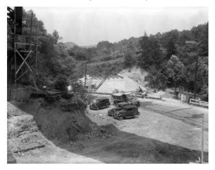
A highway underpass being constructed in a hilly, wooded area of Orange County. A crane, dump truck loaded with gravel, three cars, and workmen are also in view. Project is described with "W.P.G.H. - RC#3686". The image is a construction progress photograph taken by the Dept. of Public Works (related photograph file number 1277).
