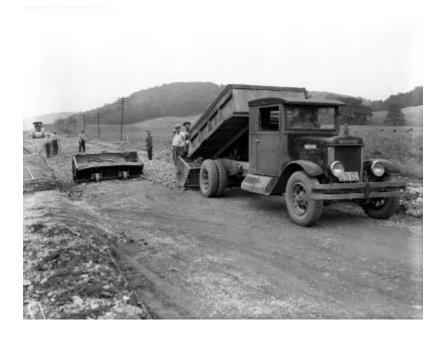
Men spreading crusher run on a road under construction in rural Cattaraugus County, possibly NYS Route 353. In the foreground, a dump truck unloads the crusher near men with shovels; in the background a man operates heavy roller equipment. Cows are on a nearby hillside. The project is associated with Public Service Commission number 6035. The image is a construction progress photograph taken by the Dept. of Public Works (related photograph file number 486).
