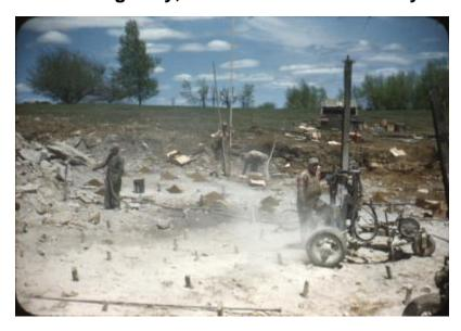
Workmen operating drilling equipment during work on state highway 8045, Broadalbin to East Galway. Image is a construction progress photograph of the Dept. of Public Works project FARC 47-64 (related photograph file no. 4644).
