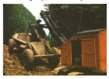
Detail of a cable shovel loading earth and rock into a bottom dump trailer. Image is a construction progress photograph of NYS Dept. of Public Works project FAS-SH47-9; Phoenicia – Stony Clove excavation (related photograph file no. 4653).
