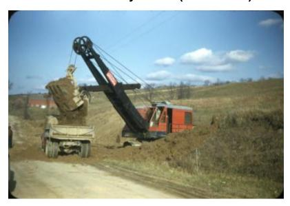
Cable shovel (Link-Belt Speeder) loading earth into a dump truck on a rural road. Image is a pre-construction photograph of NYS Dept. of Public Works project FASS 48-9, County Road Project 755; Stillwater-Schuylerville (River Road), Clarks Mills – Rensselaer County line (related photograph file no. 4810)
