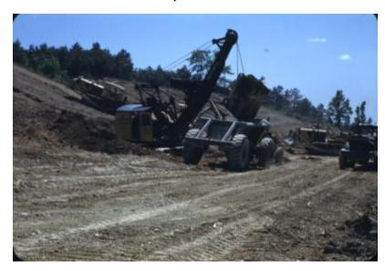
Cable shovel loading earth into a bottom dump trailer; bulldozers and other trucks also on site. Image is a construction progress photograph of NYS Dept. of Public Works project FARC 49-30, state highway 5084, Schodack Center - Valatie Road (related photograph file no. 4966).
