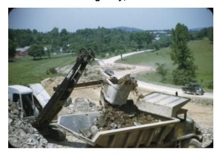
Bucyrus Erie cable shovel loading dirt and rock into a dump truck. The work site is on a roadway in a rural, hilly area. Dump truck is owned by the Lane Construction Group. Image is a construction progress photograph of NYS Dept. of Public Works project FARC 49-25 Palenville-Catskill, state highway 8231, looking west (related photograph file no. 4955).
