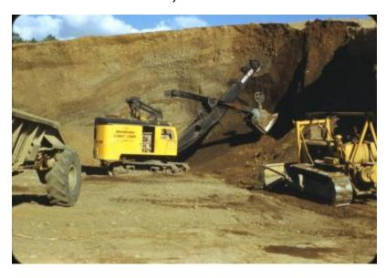
Workmen operating Northwest cable shovel, crawler tractor, and a bottom dump trailer moving earth for a highway project. The cable shovel is owned by Grandview Construction Corp., Mt. Vernon, N.Y. Image is a construction progress photograph of NYS Dept. of Public Works project FARC 49-30, state highways 5074-4, 5084-3, and 5029-2, Schodack Center - Valatie Road (related photograph file no. 5040).
