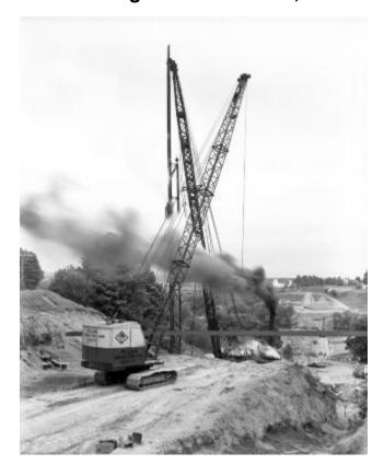
Crawler crane (owned by McLain Construction Corp., Buffalo, NY) hoisting a beam above a steam powered pile driver. The work is taking place on a hill in a rural area of Erie County. Several workmen, vehicles, other heavy equipment, a farm and farmland can be seen in the distance. The image is a construction progress photograph taken for the Dept. of Public Works (related photograph file 4300).
