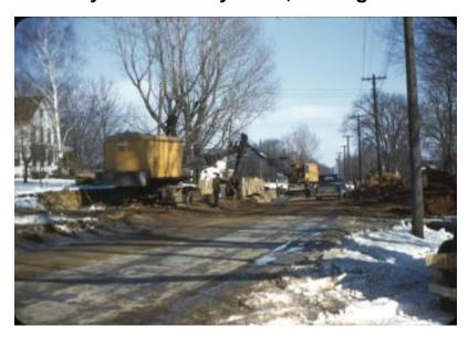
Cable shovel, crane, trucks, cars, equipment and crewmen on Troy-Schenectady Road. The road is lined with trees, telephone poles and houses. Image is part of pre-construction and construction progress photographs of NYS Dept. of Public Works project FA-RC 48-157, state highways 1, 407, and 604 Troy Schenectady Road parts 1, 2 and 3 (related photograph file no. 4878).
