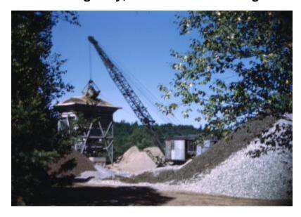
Crane and shovel loading gravel from a pile into a silo at a site in Warren County. The image is a photograph taken by the Dept. of Public Works, probably for a project on state highway 804, Luzerne - Lake George.
