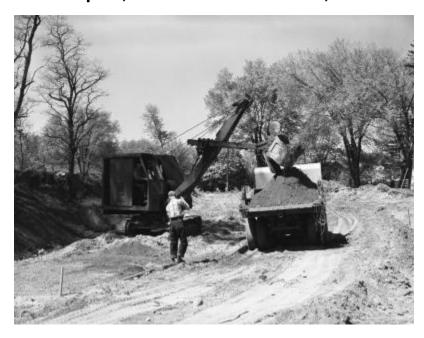
Workman operates a cable shovel loading earth in to a dump truck while another man works on the ground; part of pre-construction work on the Mohawk Turnpike in Montgomery County (NY Route 5). Trees and houses line the route under excavation. The image is a photograph taken by the Dept. Public Works (related photograph file 4470).
