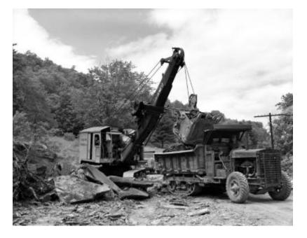
Workmen using a cable shovel, (owned by Collins Bros. of Mechanicville, NY) to load earth into a dump truck at a road construction site in a wooded area of Washington County. The image is a construction progress photograph taken by the Dept. of Public Works (related photograph file 4480).
