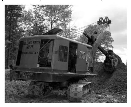
Workman operating a Bucyrus Erie cable shovel (owned by Collins Bros. of Mechanicville, NY) while another workman looks on at a road construction site in Washington County. The image is a construction progress photograph taken by the Dept. of Public Works (related photograph file 4480).
