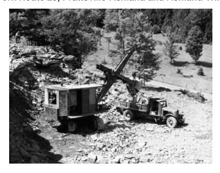
Bucyrus Erie cable shovel loading rock into a dump truck; a workman watches from a rocky hill. The work is for construction of NY Route 23, State highways 5491, Prattsville-Ashland and SH 8051, Ashland-Windham. The image is a construction progress photograph taken by the Dept. of Public Works, (related photograph file number 4500).
