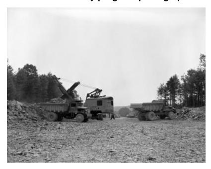
Crawler cable shovel (owned by N.R. Corbisello of Binghamton, NY) loads rock into dump trucks during Catskill Thruway construction. The work is probably in Greene County. Background includes woods, workmen, trucks, and construction equipment. The image is a construction progress photograph taken by the Dept. of Public Works, (related photograph file number 4511).
