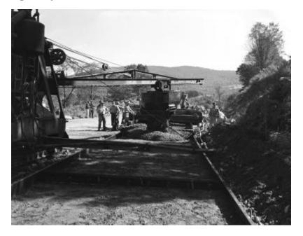
Paving crew and equipment spreading crusher during construction of state highway 615 (NY 20) New Lebanon to Brainard and state highway 5108 (NY 20) in Brainard Station; a policeman looks on in the background. The image is a construction progress photograph taken by the Dept. of Public Works (related photograph file number 4530).
