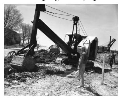
Workmen and two cable shovels, one owned by Lancaster Corp., Meriden Conn., excavating for state highways 5569 (NY 145/US 20) Sharon to Sharon Springs. Several trucks and a barn are also in view. The image is a construction progress photograph taken by the Dept. of Public Works, Bureau of Highways (related photograph file number 4637).
