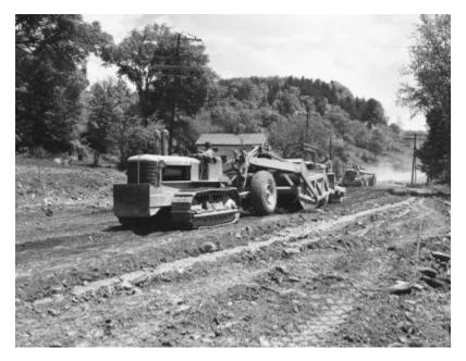
Workmen operate crawler tractors and scrapers during road construction of NY Route 23, State highways 5491, Prattsville-Ashland and SH 8051, Ashland-Windham. A small house, truck and woods are also in view. The image is a construction progress photograph taken by the Dept. of Public Works, Bureau of Highways (related photograph file number 4654).
