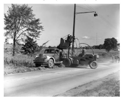
Workman operating a Wagner Scoopmobile dumps grass and dirt into a NYS Dept. of Public Works truck. Three men follow the vehicles brushing debris off the highway. The area is rural, a barn and what might be radio antennas are also in view. The image is a construction progress photograph taken by the Dept. of Public Works (related photograph file number 4766).
