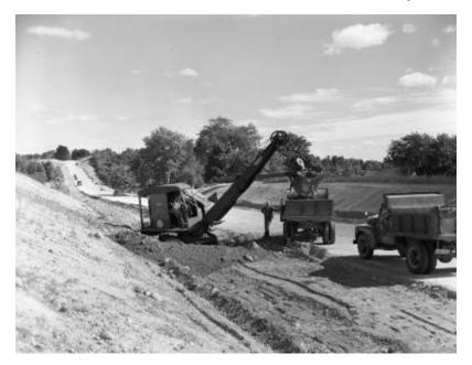
Bucyrus Erie cable shovel loading rock and earth into dump trucks alongside a state highway in a rural area of Saratoga County (SH 8045). Several cars and trucks travel on the road nearby. The image is a construction progress photograph taken by the Dept. of Public Works (related photograph file number 4767).
