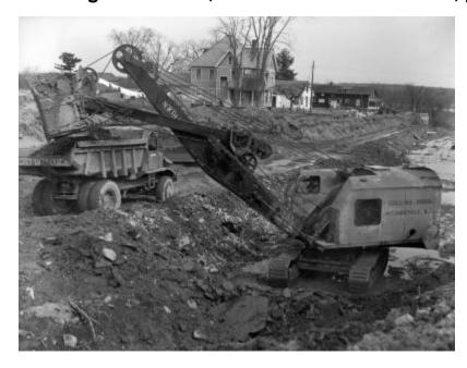
Northwest cable shovel, owned by Collins Bros., Mechanicville, N.Y., loading dirt into a dump truck at an excavation site. The image is a construction progress photograph taken by the Dept. of Public Works, Bureau of Bridges and Grade Crossings (related photograph file number 4873).
