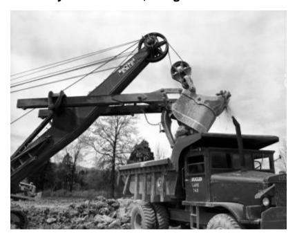
Detail of a Bucyrus Erie cable shovel loading earth in to a dump truck in a wooded area. A bulldozer can be seen in the background. The image is a construction progress photograph taken by the Dept. of Public Works, Bureau of Public Relations (related photograph file number 4929).
