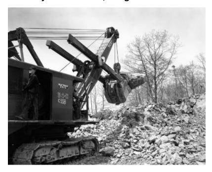
Detail of workman operating a Bucyrus Erie cable shovel loaded with rock; a second workman stands on the shovel's platform. The image is a construction progress photograph taken by the Dept. of Public Works, Bureau of Public Relations (related photograph file number 4929).
