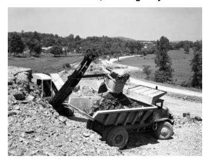
Detail of a Bucyrus Erie cable shovel loading earth into a dump truck owned by Lane Construction Corp., Meriden, Conn. The work site is off a winding road in a rural area; farms are also in view. The image is a construction progress photograph taken by the Dept. of Public Works, Bureau of Highways, (related photograph file number 4955).
