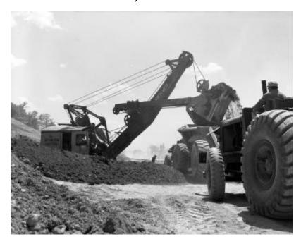
Detail of a Northwest cable shovel, owned by Grandview Construction Corp., Mt. Vernon, NY, loading earth into bottom dump trucks. The image is a construction progress photograph taken by the Dept. of Public Works, Bureau of Highways (related photograph file number 4966).
